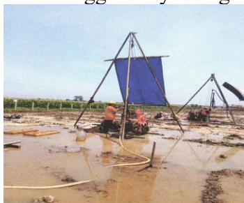
Figure 6. Coring work for test specimen sampling
