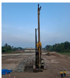
(a) PT Keller Ground Indonesia
